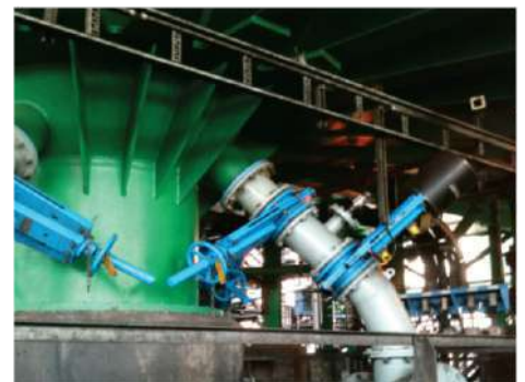
Coal Washing Plant
